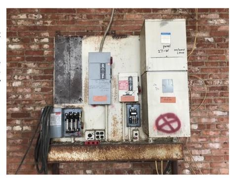
**Covering:** Energized panels must cover to prevent contact with live electrical parts. If a licensed electrician is actively working on the panel the cover may be removed. It is the responsibility of the electrical contractor to protect themselves and the other subs from electrical hazards All spaces on the panel must be covered by a breaker or a cover to prevent contact with energized components.
